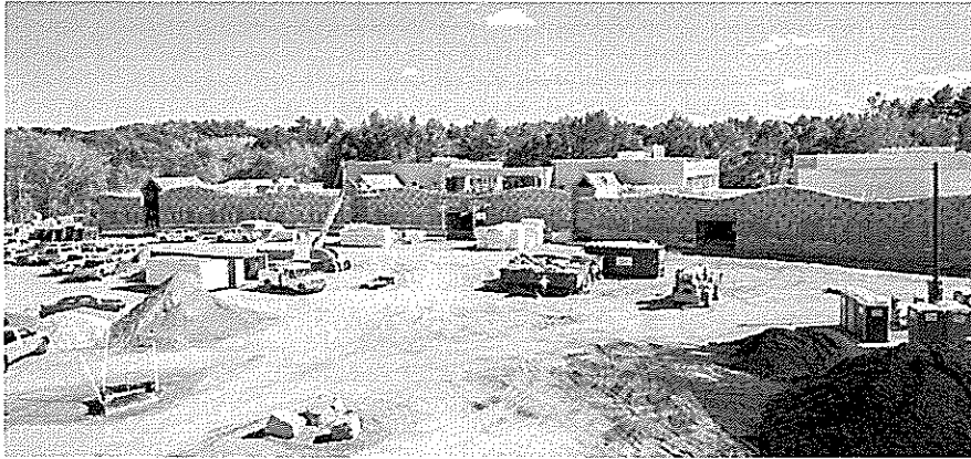
Full Building Front
